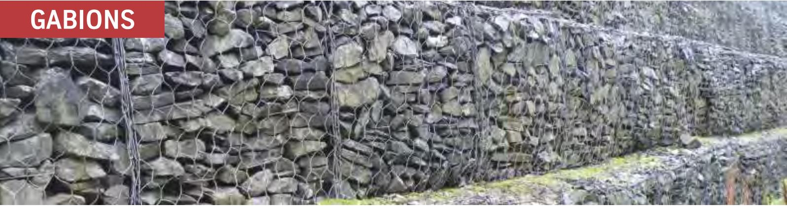
Gabions are rectangular wire mesh baskets filled with rock at the project site to form flexible, permeable, monolithic structures such as retaining walls for commercial, industrial and road projects. Gabion and Gabion mattresses are trusted, well proven and technically sound solutions to retain earth and reduce erosion. This technique is extensively used around the world. They are also used for river bank stabilization, channel linings and weirs.
