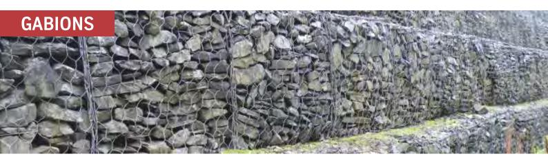
Gabions are rectangular wire mesh baskets filled with rock at the project site to form flexible, permeable, monolithic structures such as retaining walls for commercial, industrial and road projects. Gabion and Gabion mattresses are trusted, well proven and technically sound solutions to retain earth and reduce erosion. This technique is extensively used around the world. They are also used for river bank stabilization, channel linings and weirs.
